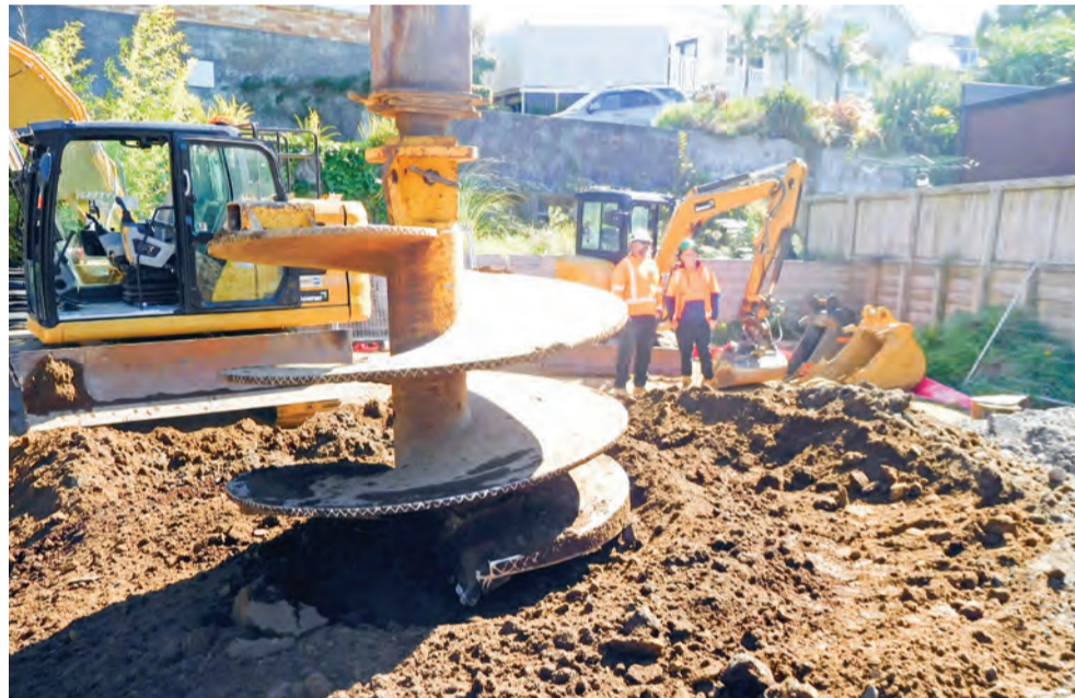
Big gear tackles the big job of repairing the Waiwaka Terrace culvert.
